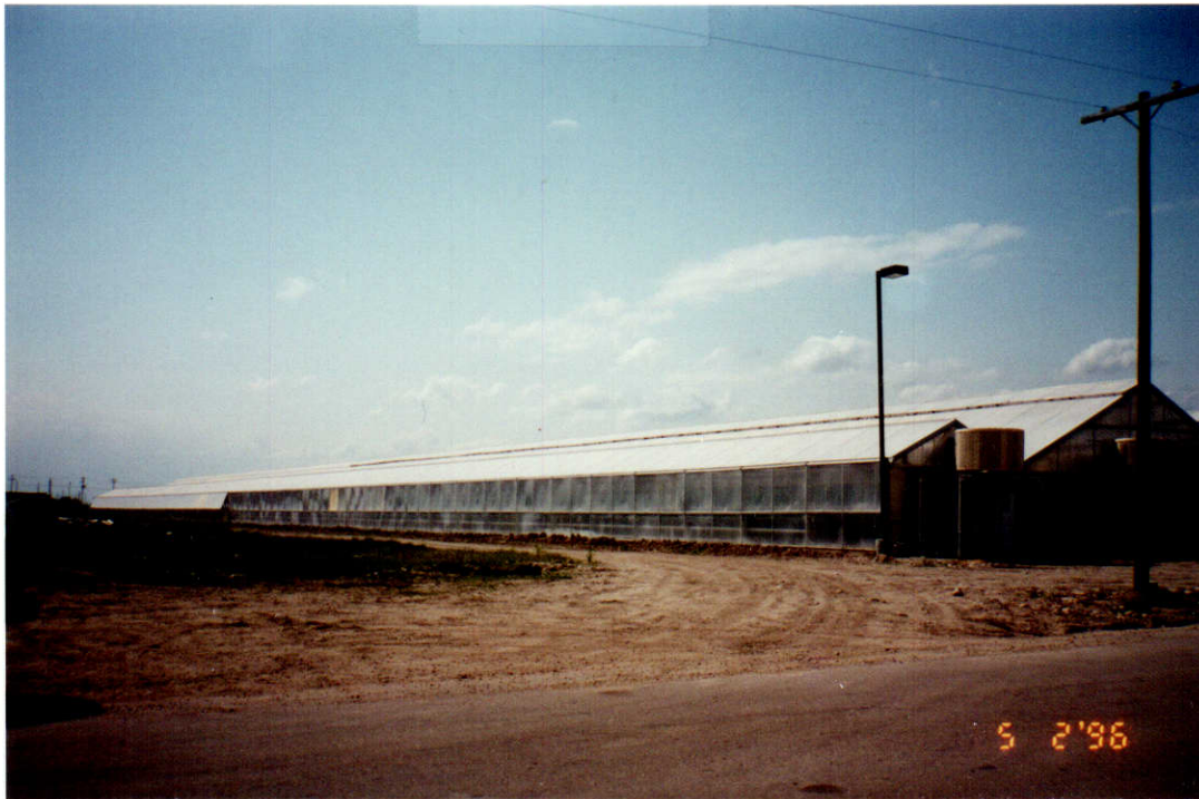
Primary House - (Cooling system visible end of building - see 10629)
