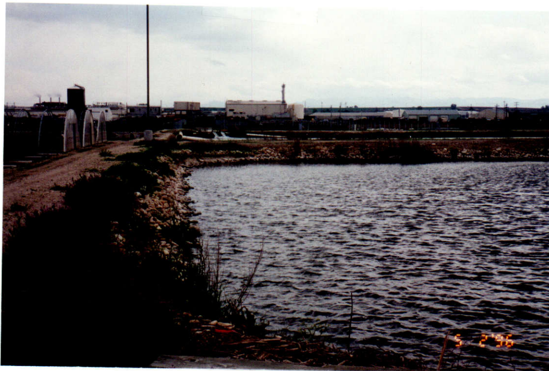
Lagoon/ Discharge Cooling Pond
