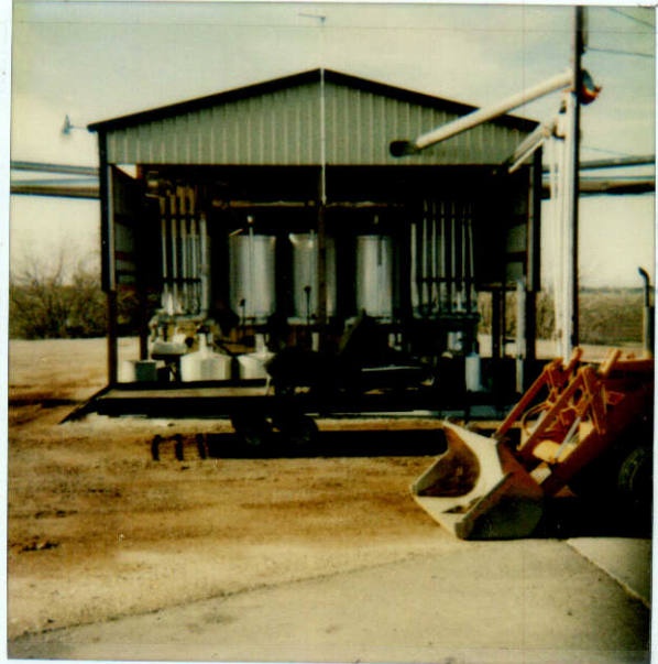
STEAM TANKS FOR STILL
