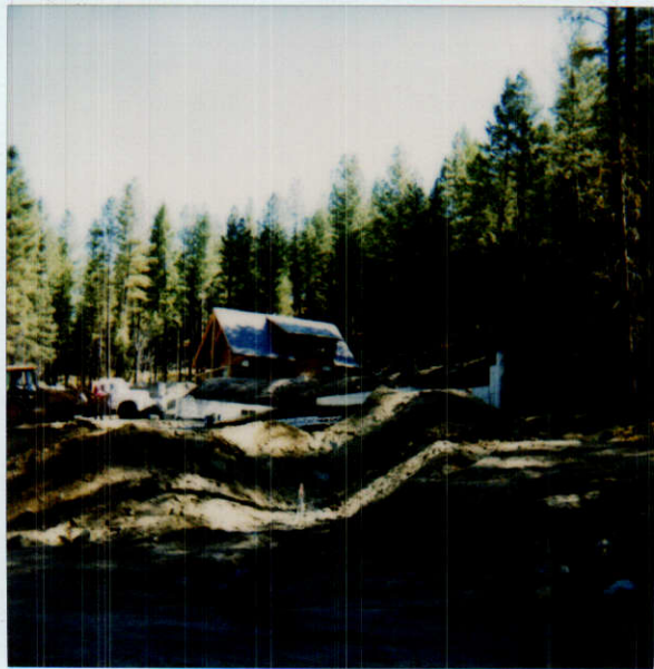
NEW CONSTRUCTION WITH EXISTING HOME (IN REAR) PARADISE SUBDIVISION
