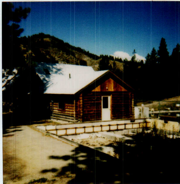
Cabin and Foundation (East of Lodge) Lot 38
