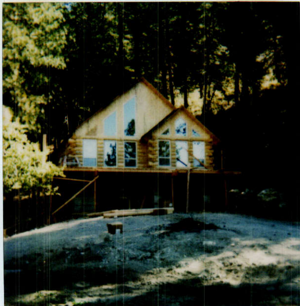
Home Under Construction Paradise Subdivision
