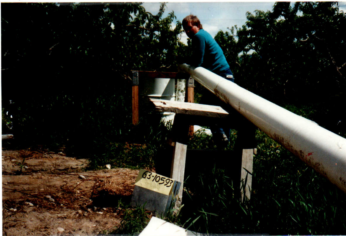
MEASUREMENT LOCATION AND P/U PICTURE # 2 LOOKING SOUTH EAST.
