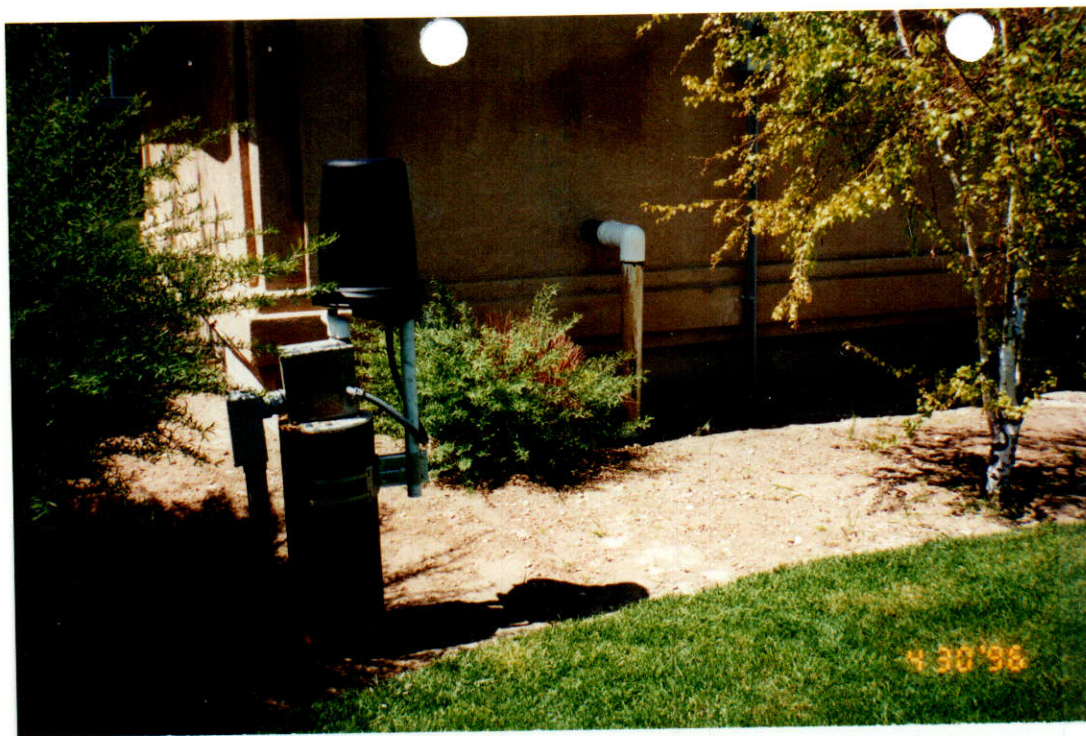
P/O View to NW Pumphouse in background
