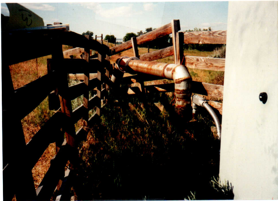
#6. Irrigation well site and casing with 5" discharge pipe to a buried 5" mainline.
