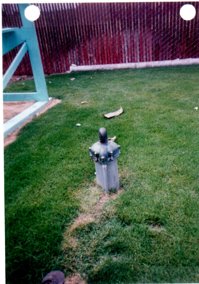
View of casing. This well is located on the south side of the property.
