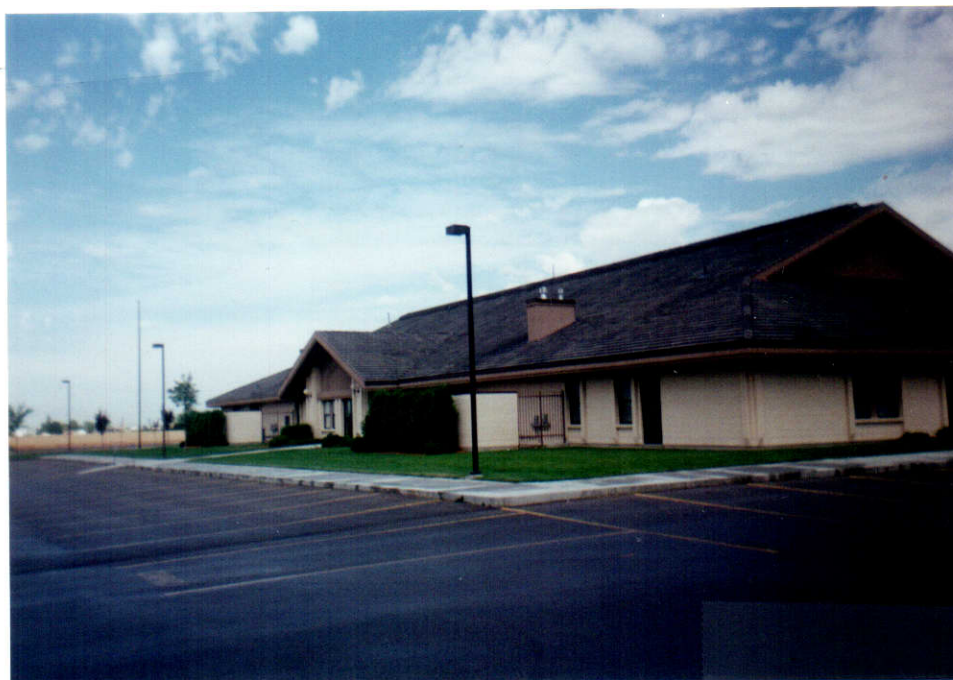
View of Church. Line from well goes into line underground lawn is planted with pop-ups
