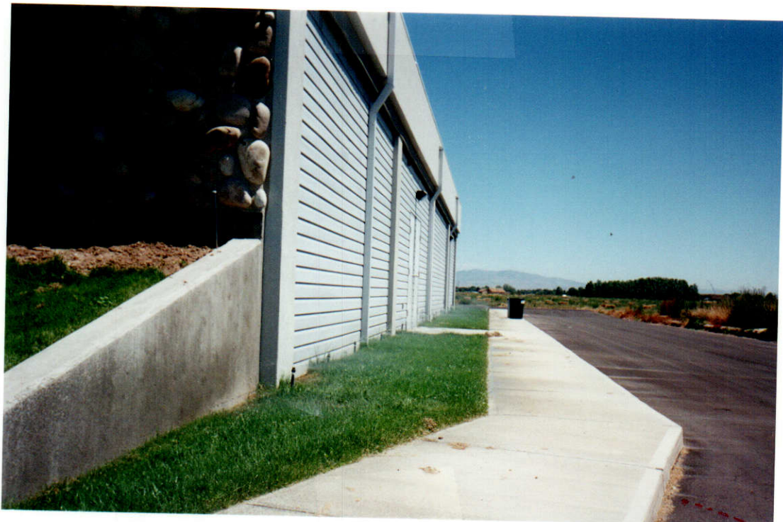
PHOTO FOUR- Underground sprinkling system in operation, south side of church.
