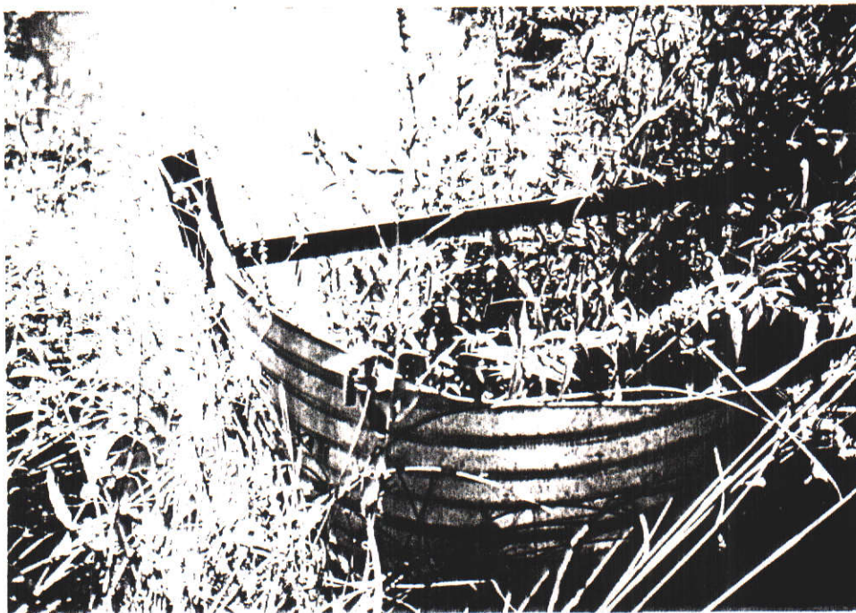
VIEW OF HEADGATE. FROM THIS STRUCTURE WATER MAY BE LET OUT OF THE CANAL / MARSH TO BE SPILT IN DIXIE SLOUGH.
