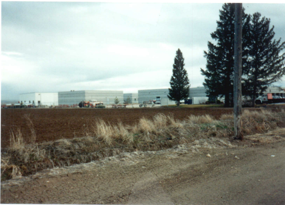
#10 View of the shop, storage and office/research building looking Northeast from Hwy 20/26.
