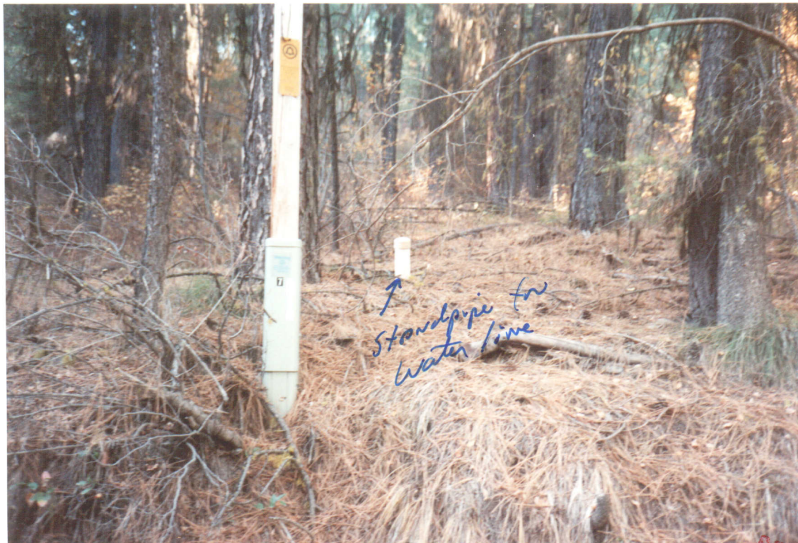
PHOTO TWO- Standpipe for stubbed line on Lot 14 next to well.
