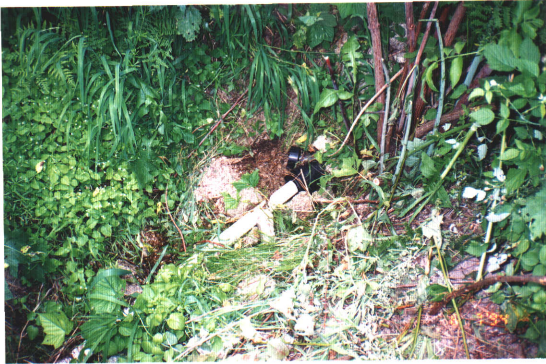
P/D Showings Connection & overflow valve
