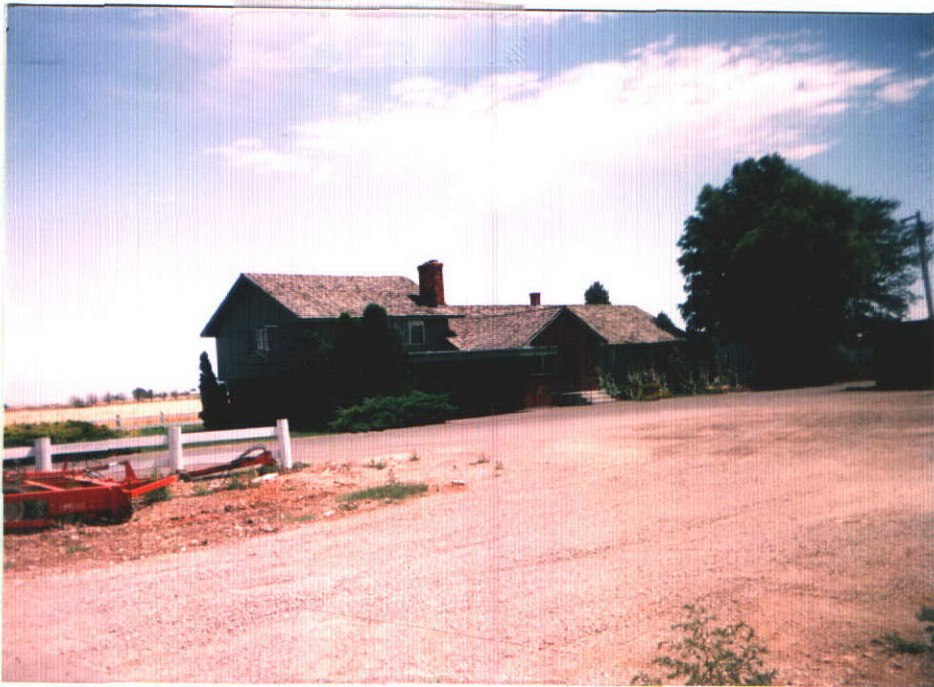
view of house from the north side of property.
