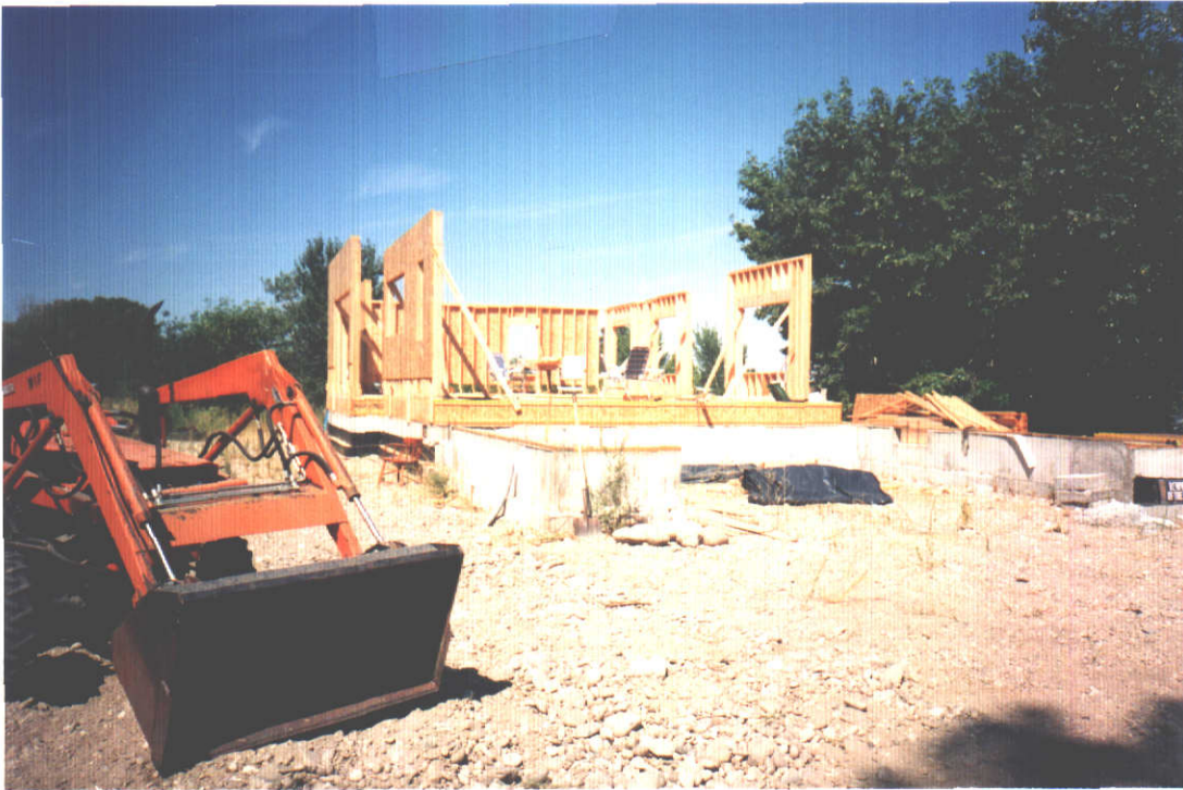
house being built on property (97.5' x 90')
