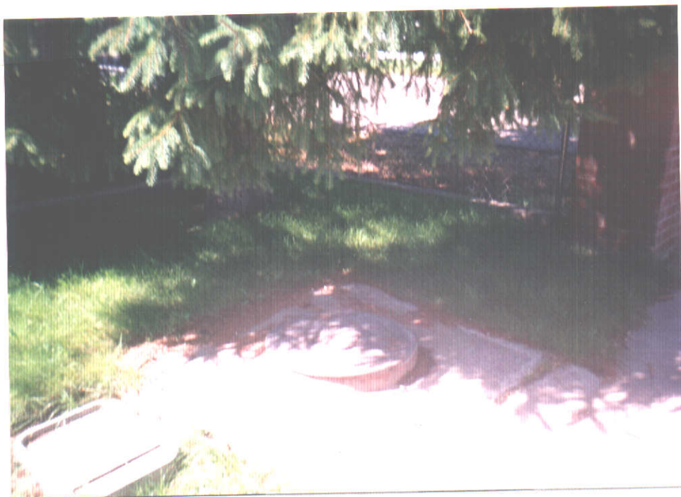
View of well housing. Well is under this iron top. This casing is the well is located in the S/W corner of the lawn.
