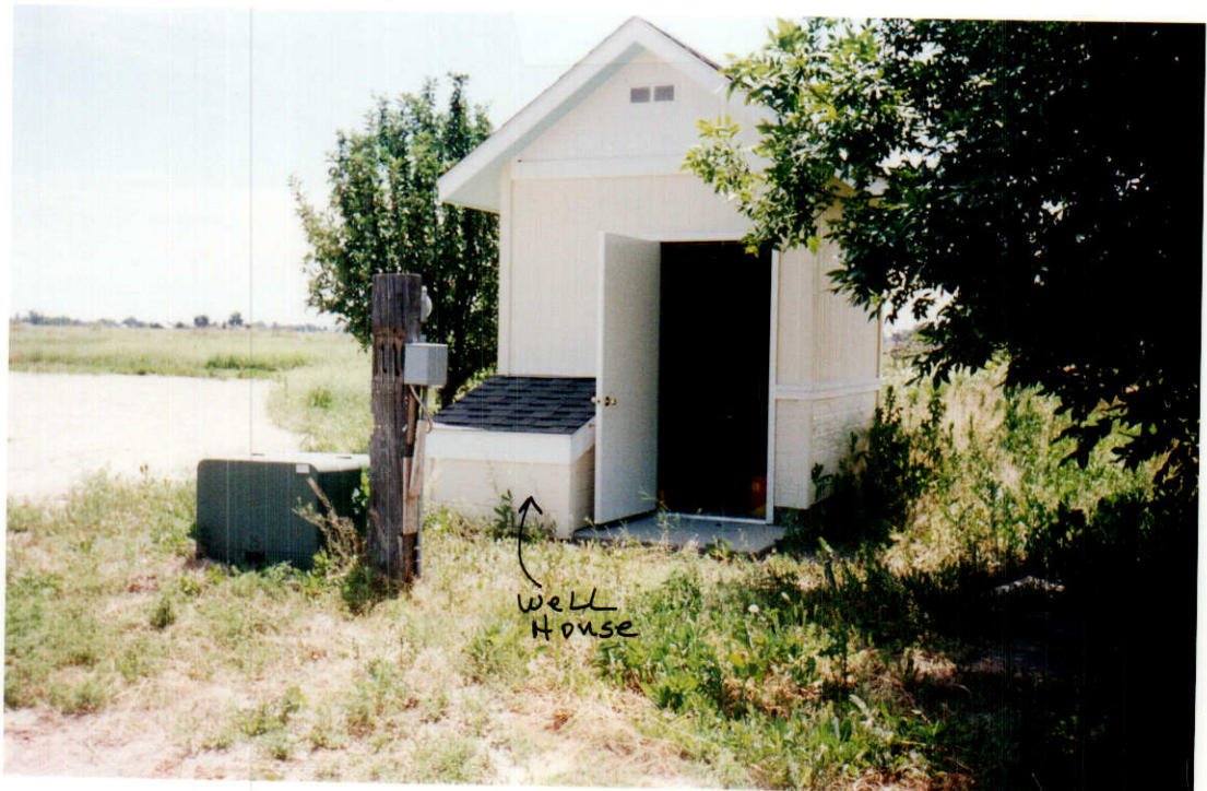
PHOTO TWO- Pump house and well house (small structure on end).
