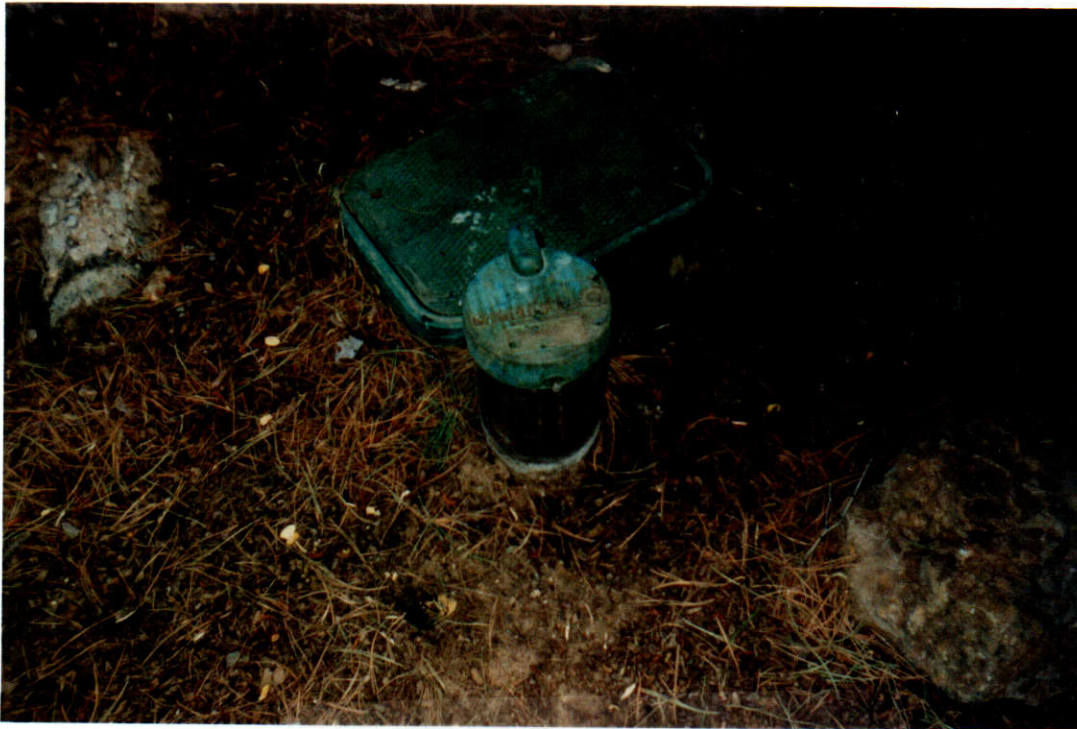
view of well casing located in front of house @ West/North part of property
