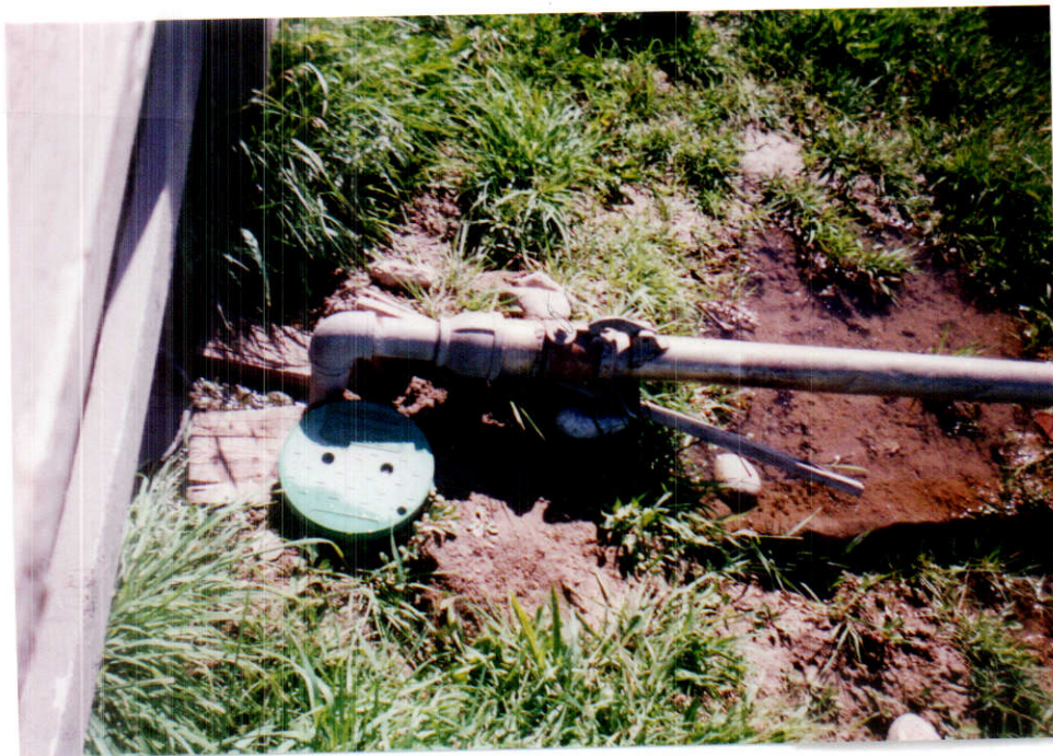
THE PASTURE IS IRRIGATED WITH THIS TYPE OF CONVEYANCE SYSTEM. THIS RISER WITH ALUMINUM PIPE IRRIGATES THE PASTURE.
