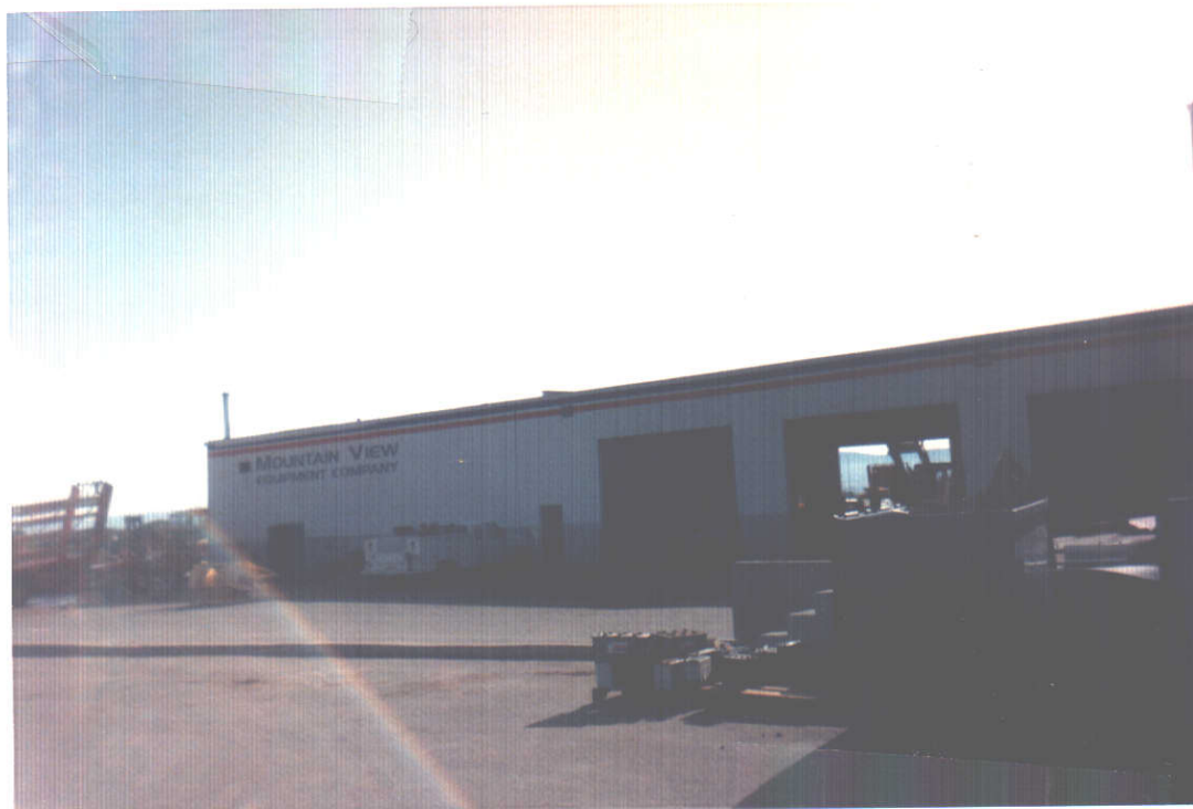
View of the "shop". Located in the northern portion of property.
