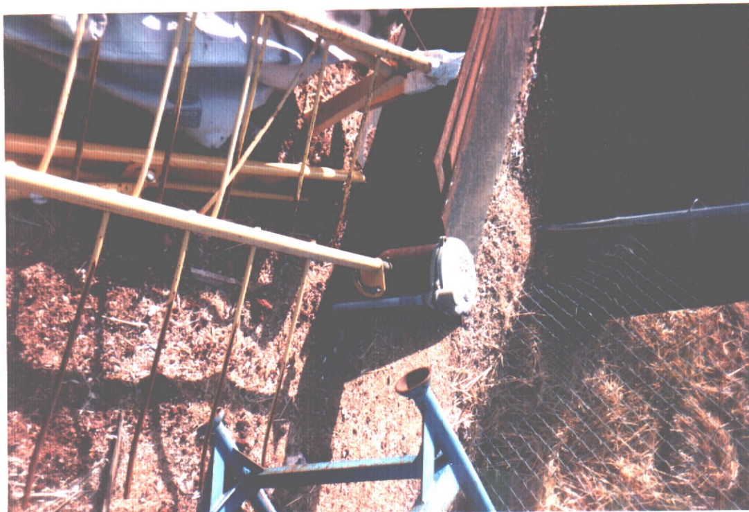
View of well: Located AT THE WEST SIDE OF PROPERTY.
