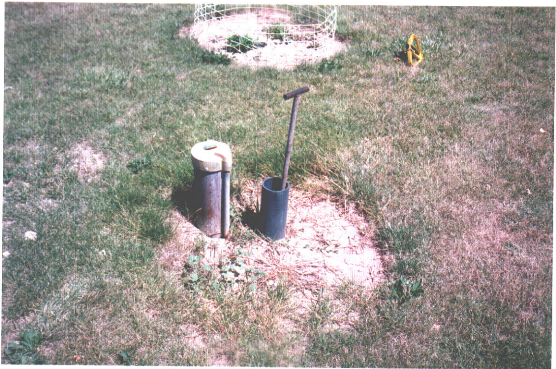
PHOTO ONE- Well and control valve located in front yard.
