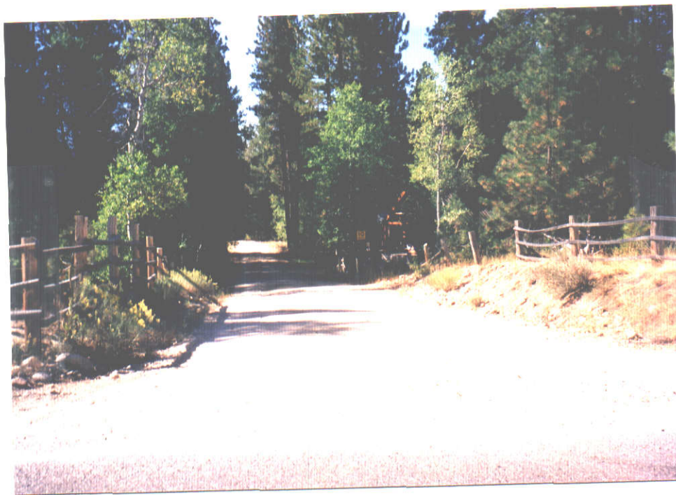
Place of use from main road looking South toward River Drive 17 2000
