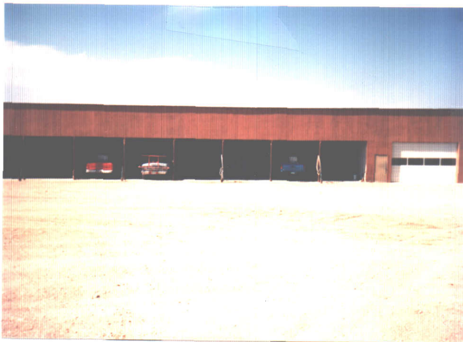
#7. Storage shed for spray trucks. belonging to county weed control district.
