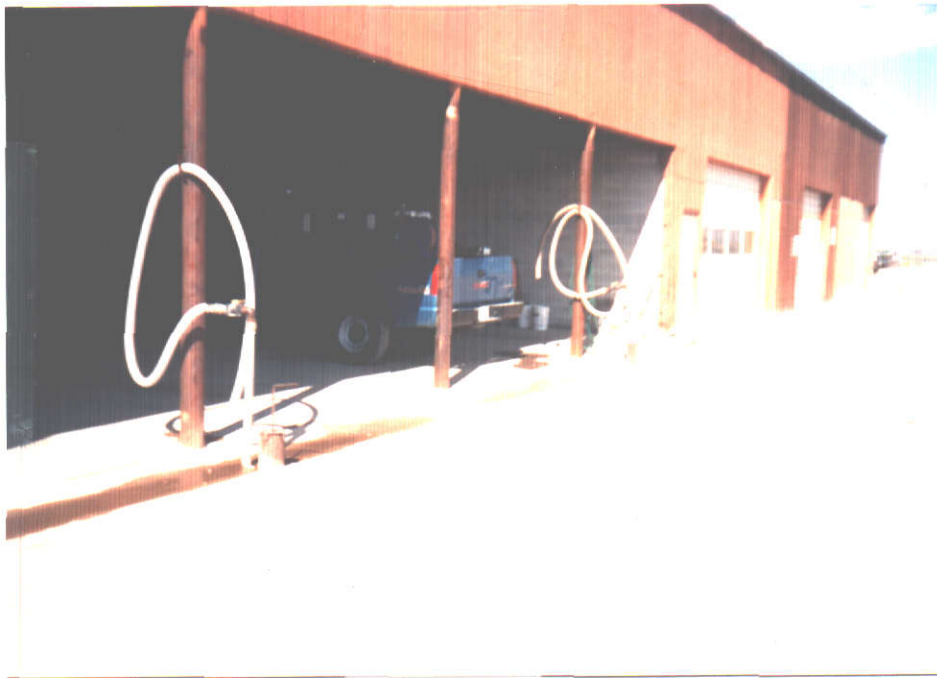
#8. Hydrants and hoses used to fill spray truck tanks
