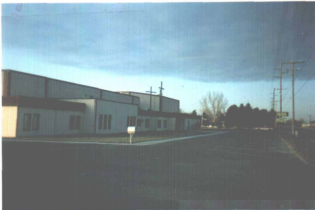
View NW. view of front IRRIGATED LAWN & IRRIGATED STRIP.
