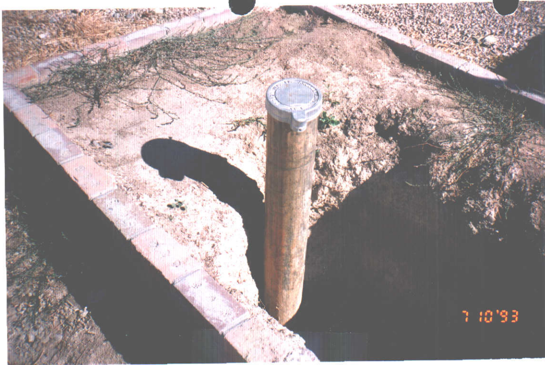
6" well - no pump
