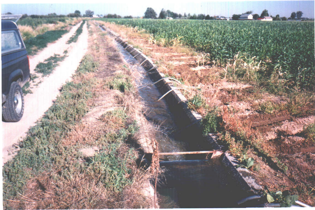
PHOTO THREE- View westerly of concrete ditch and siphon Tubes used To irrigate corn field. A cipolletti weir is shown installed in concrete ditch.
