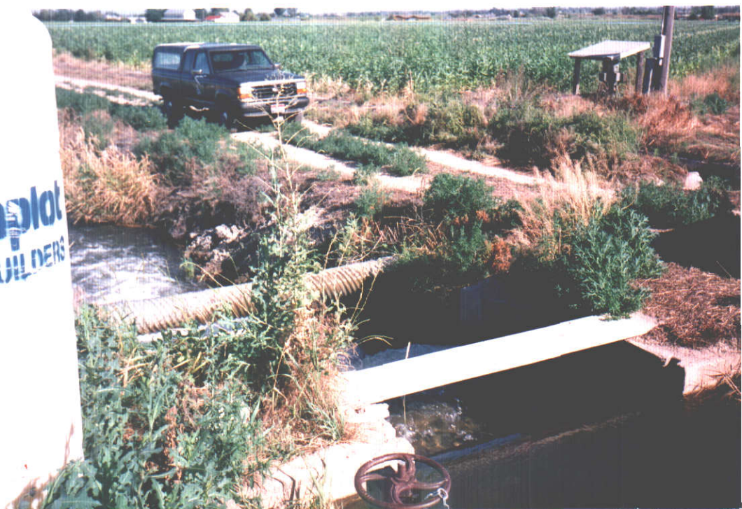
PHOTO FOUR- View northwest of CMP crossing Fogarty Lateral. Pipe connects concrete ditch to irrigation box on south side of Lateral.
