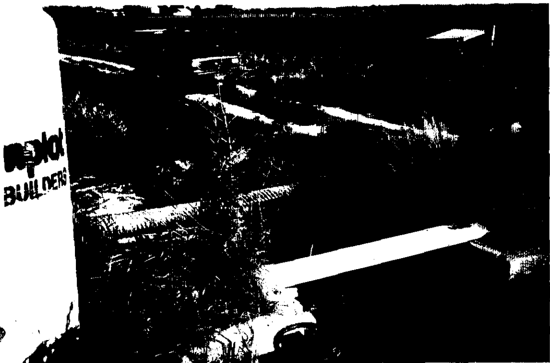
PHOTO FOUR- View northwest of CMP crossing Fogarty Lateral. Pipe connects concrete ditch to irrigation box on north side of lateral.
