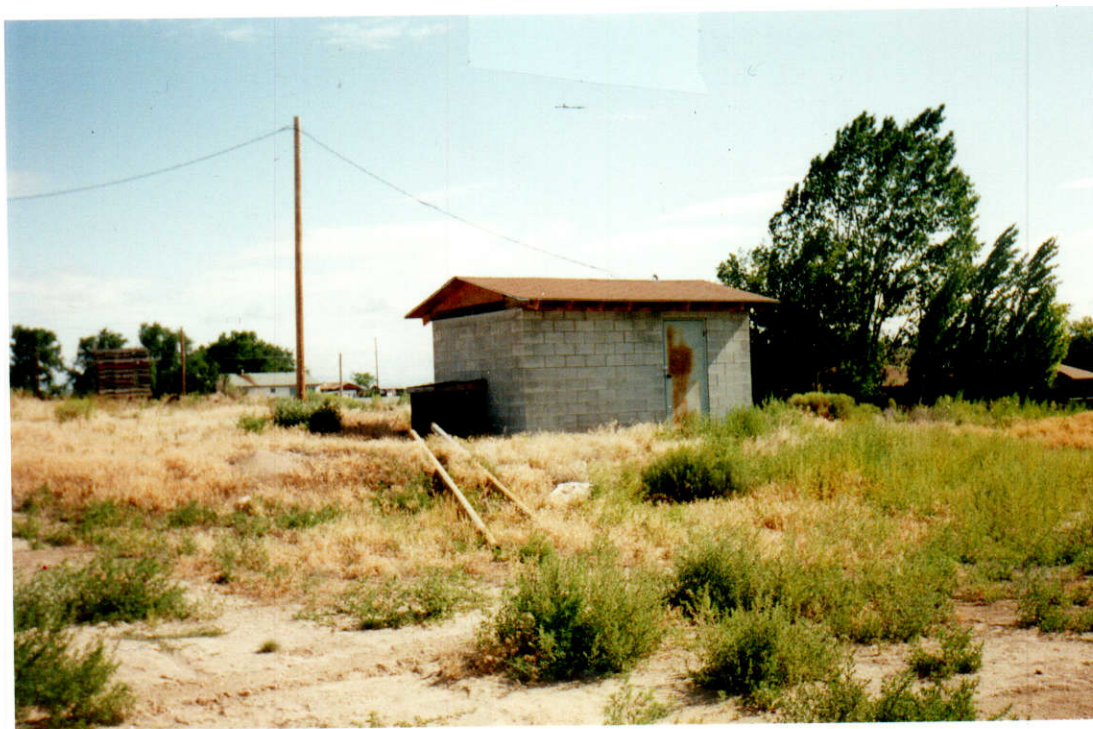
PHOTO ONE- well / Pump house located near (northeast) ? corner of development. Well is enclosed by small structure next to large building. Large building contains 1500 gallon Pressure Tank.
