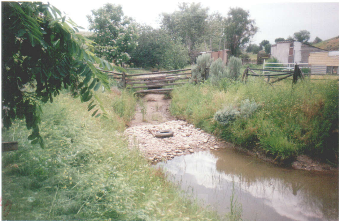
PHOTO EIGHT TWO View southward of dam spillway or overflow.
