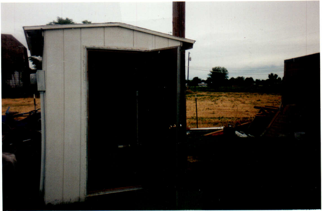
PHOTO ONE- Well And Pump House Located near north end OF mobile Home Court.
