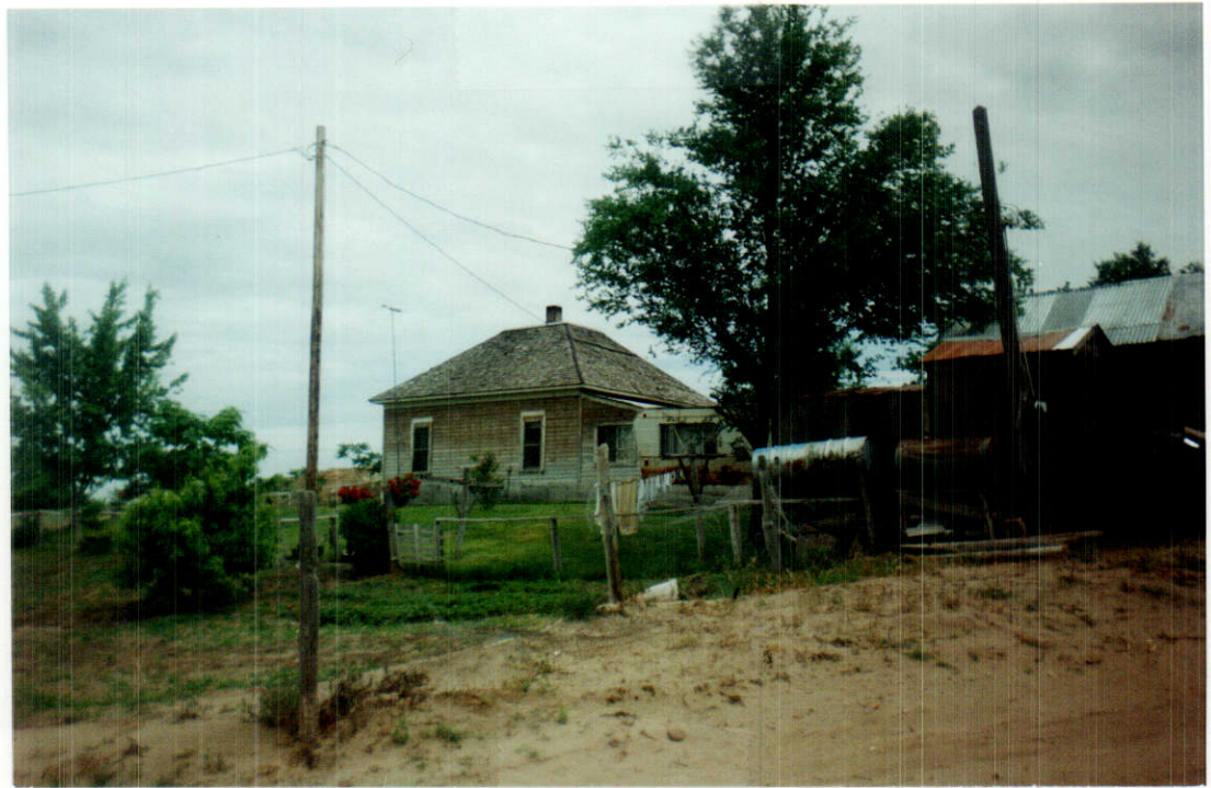
PHOTO THREE- View northeast of home. Well house is shown to the right side of photo.
