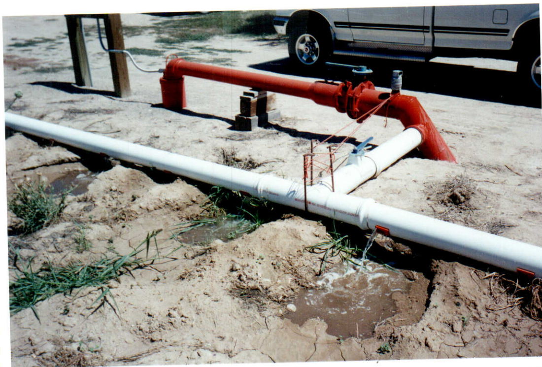
PHOTO ONE- Well And gated pipe, 6", discharging into onion field.
