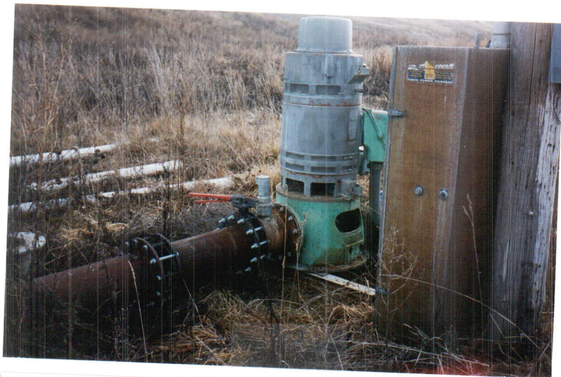
View southeast of well No. 2.
