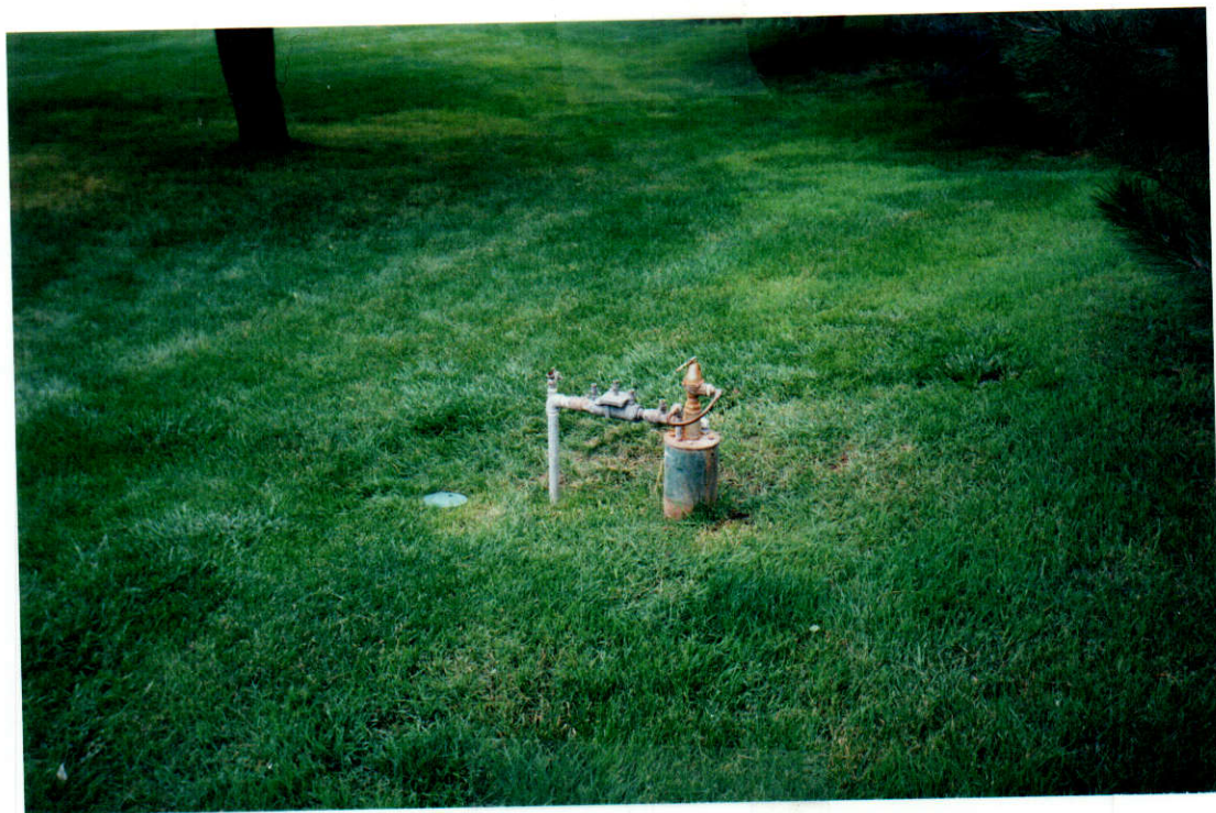
PHOTO ONE- Well and underground sprinkling system. Well is located in back yard near southern property line.
