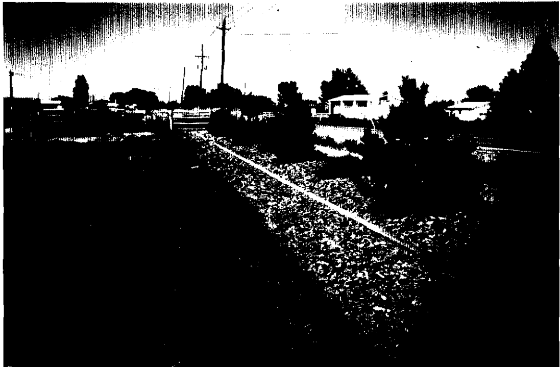
PHOTO THREE- View northwesterly OF 4" main Line. Pipe is hooked To riser and connected to gated pipe in pasture.
