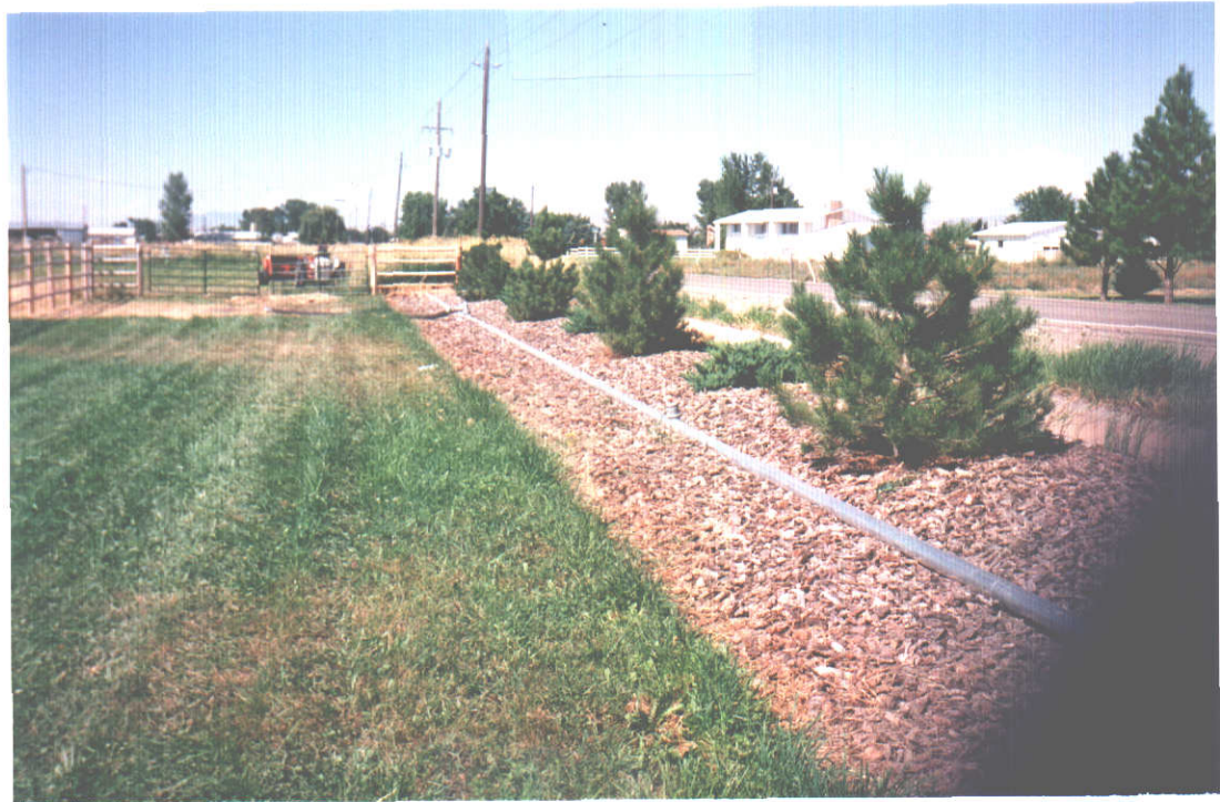
PHOTO THREE- View northerly of 4" main line. Pipe is hooked to riser and connected to gated pipe in pasture.
