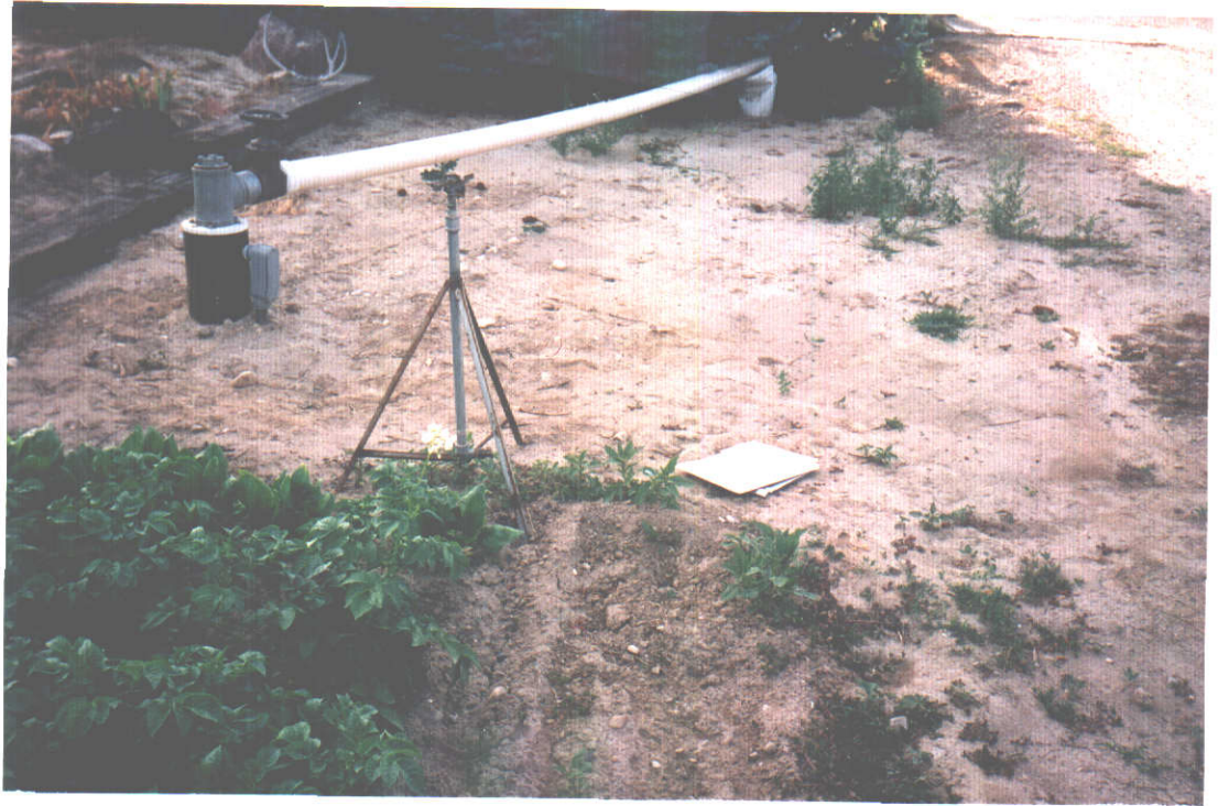
PHOTO THREE- Well and 4" PVC Leading to and Terminating at concrete irrigation ditch.
