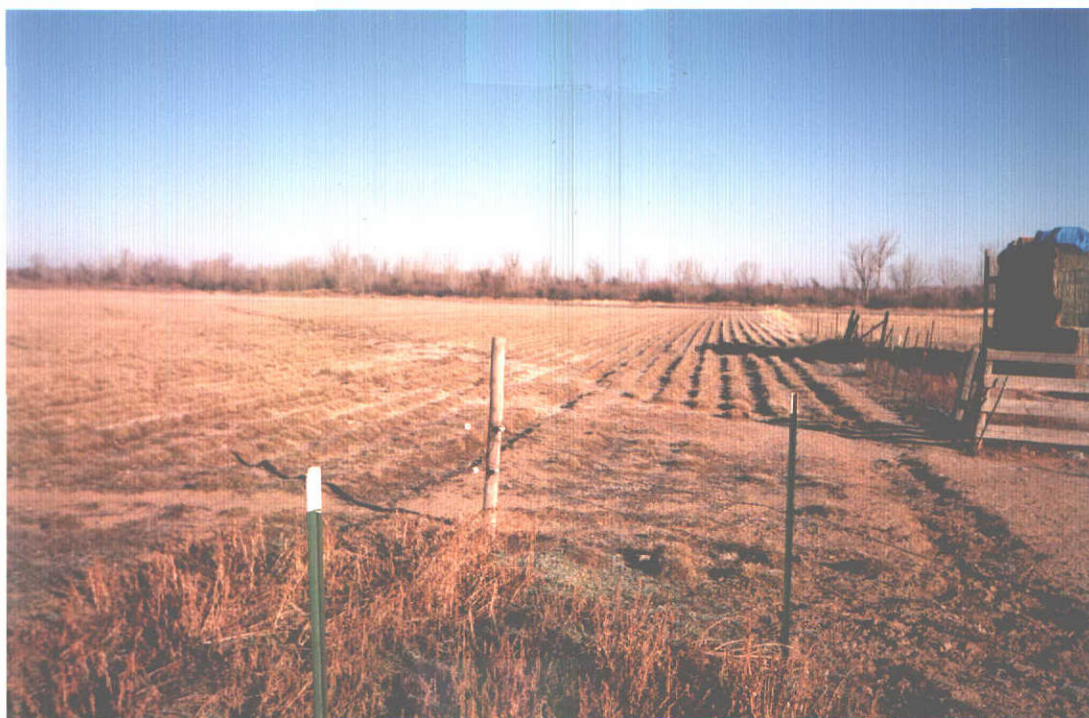
PHOTO THREE- View northerly of EAST end of Field and west end of pasture. Buried 6" PVC surfaces in corner of pasture and is connected to irrigation pipe for irrigation.
