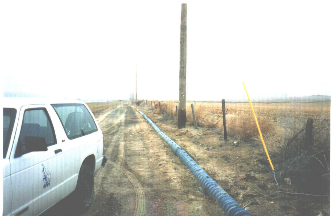
PHOTO FOUR- View west of plastic pipe delivering water to irrigation ditch.
