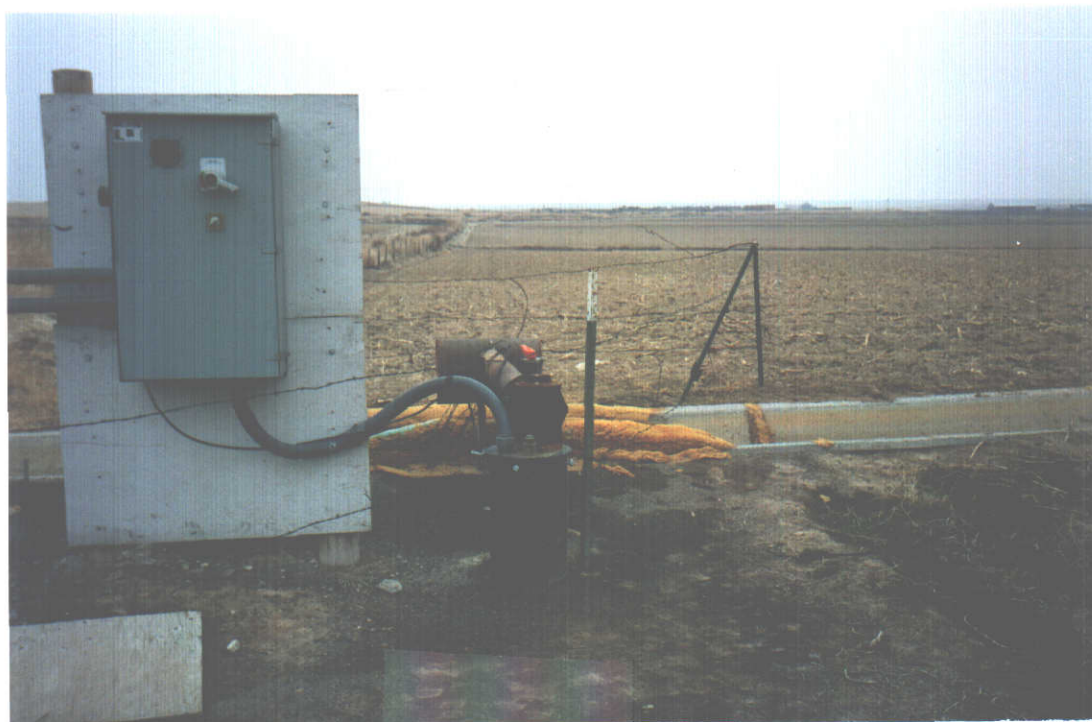
PHOTO ONE- Well and portion of acreage to the east of well. Water is discharged in concrete ditch and distributed to the south and west.
