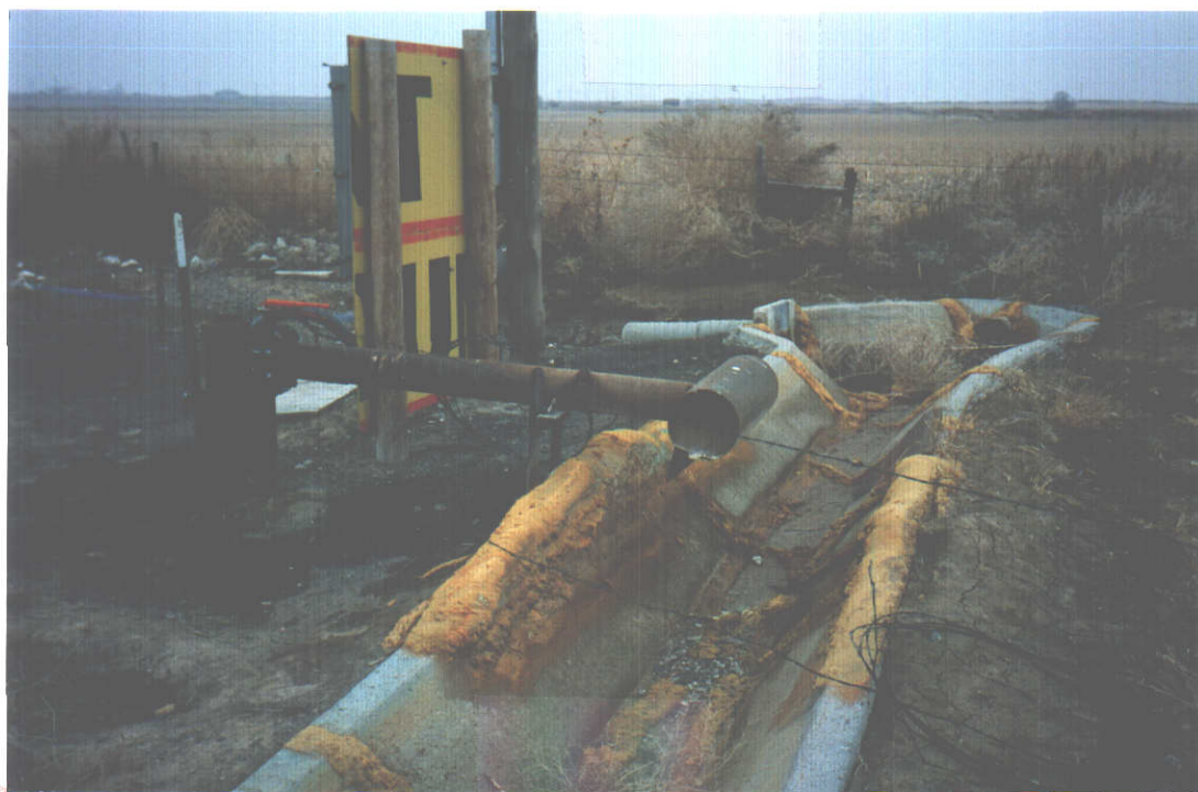
View north of discharge line and concrete ditch. Water is piped to the west to irrigation ditch.
