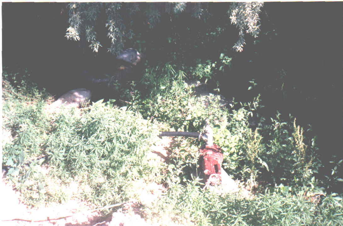
P/O & diversion dam in Hellyer drain
