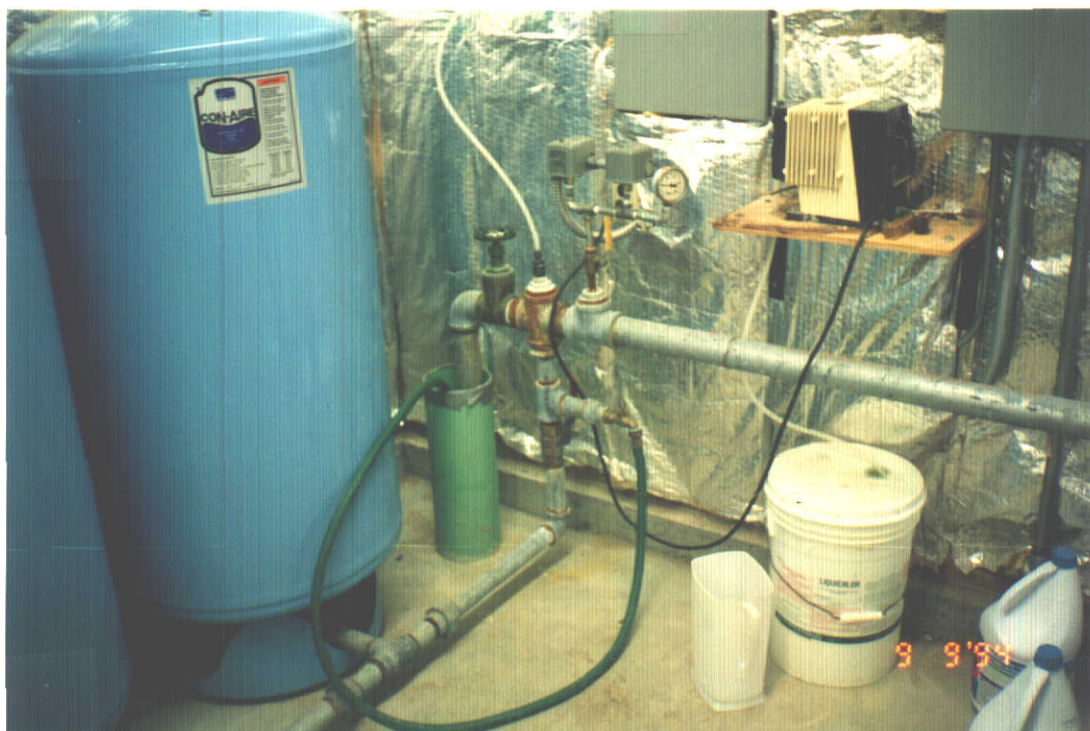
Chlorination point & pressure system for 5 new homes
