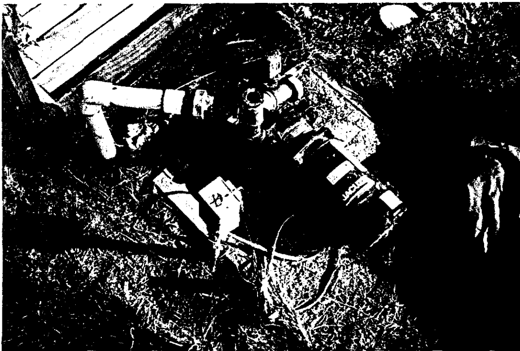
1 HP GE MOTOR JACUZZI PUMP ARTESIAN WELL
