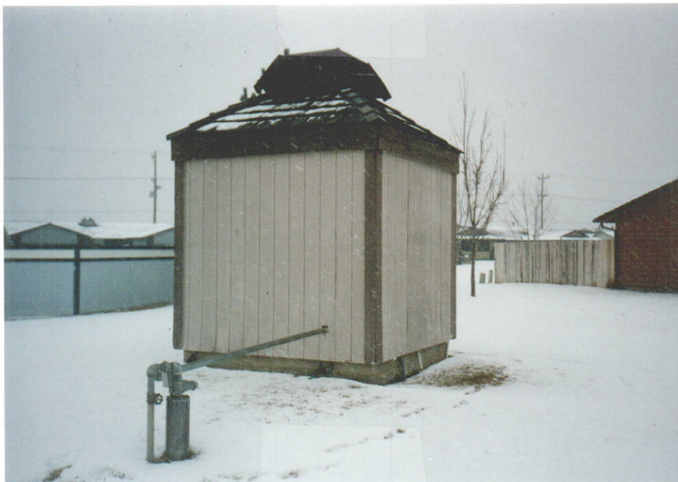
view easterly of well and pump house.
