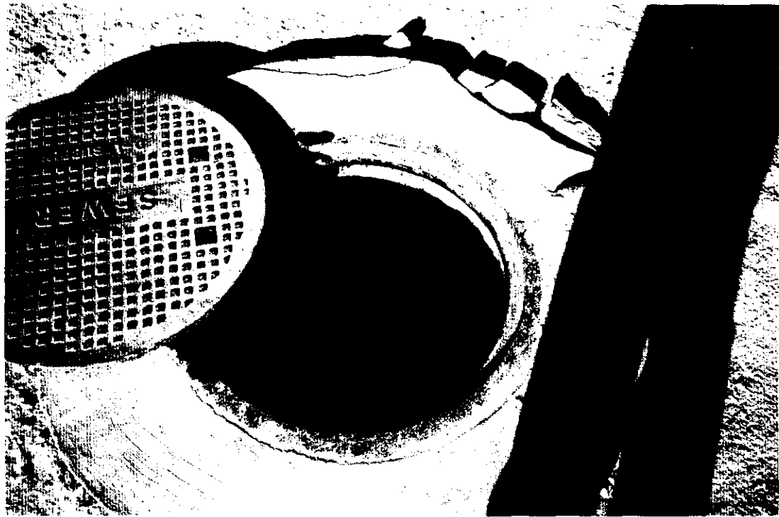
PHOTO ONE- well located in 3' diameter concrete manhole.
