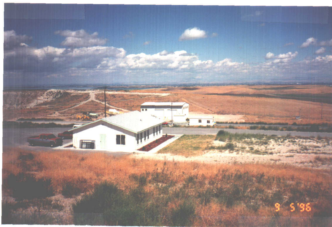
P/u office in foreground, scale house Right of Center, Public restrooms Center, Shop in background. View looking North
