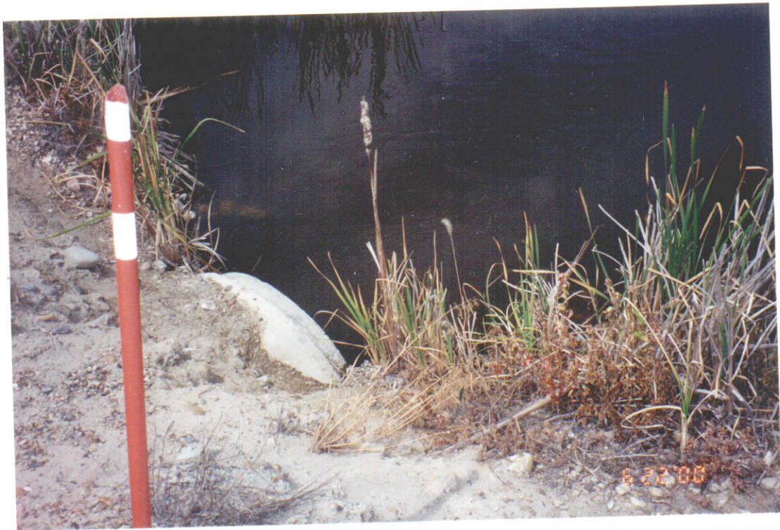
Point of diversion
