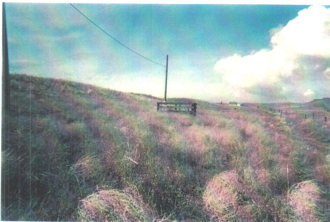
Irrigation Well #2- Viewed looking to the northwest
