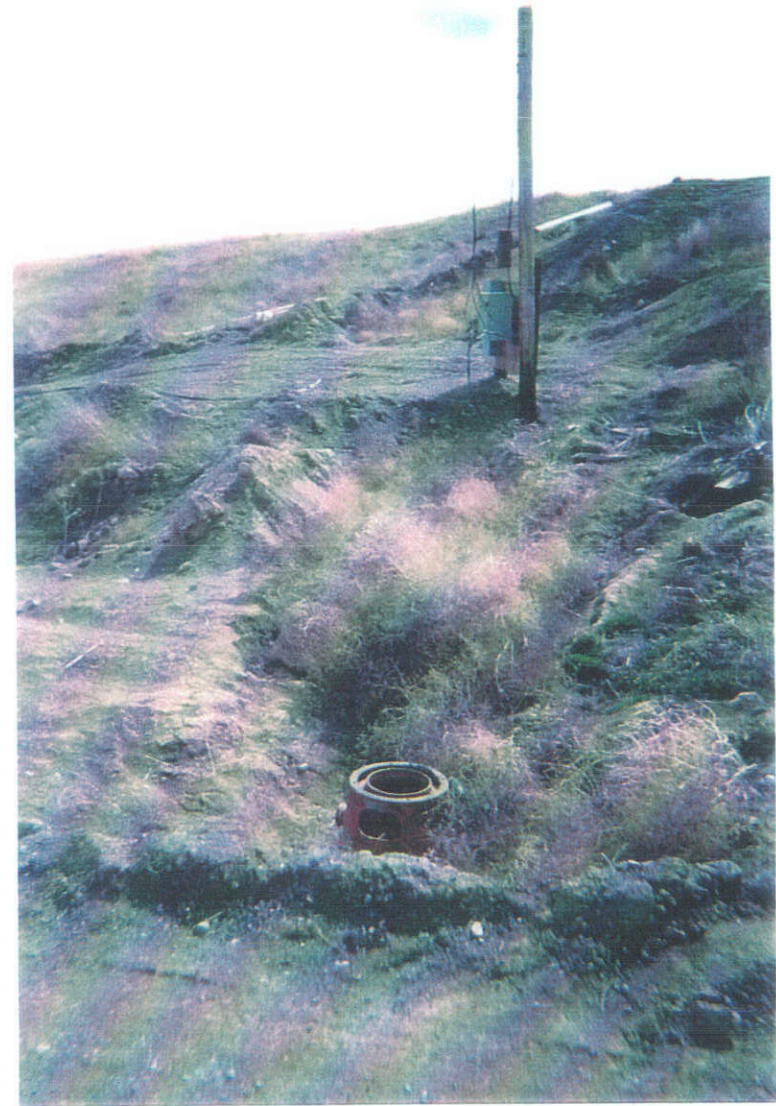
Irrigation Well #1- Viewed looking south Irrigation pipe and trench in background
