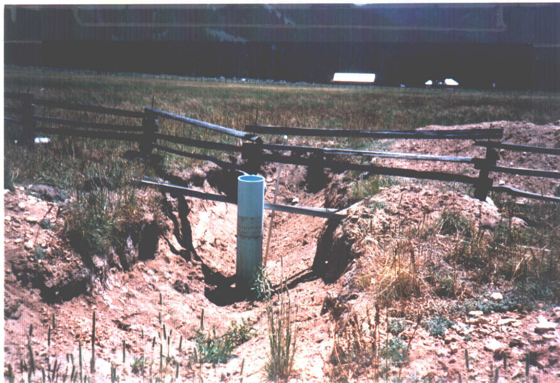
RISER AT EDGE OF PASTURE.
