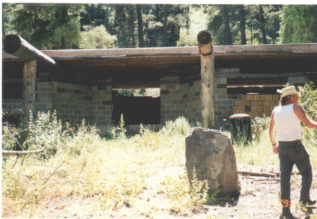
pk under construction
