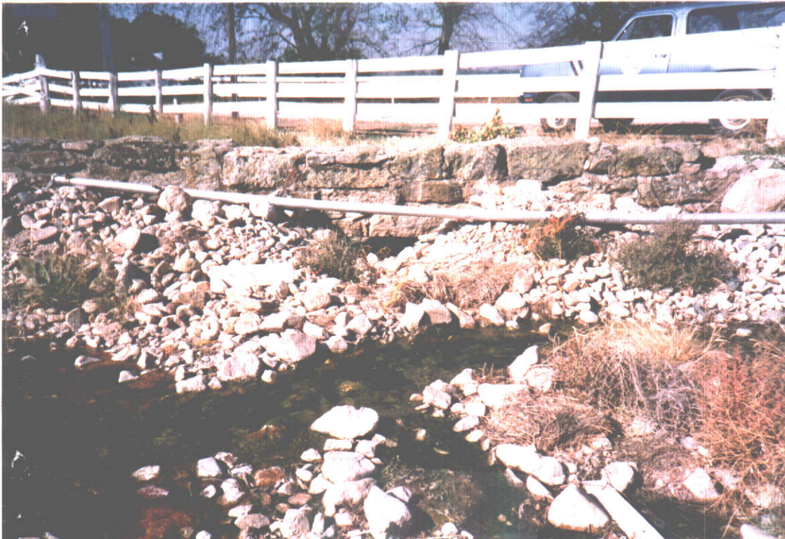
Rediversion point A from Warm Springs Creek to P.U.
