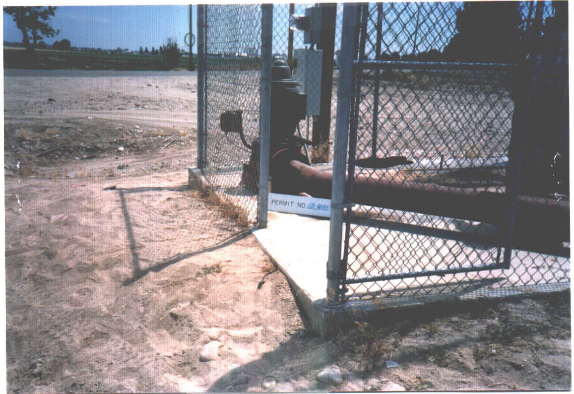
Point of Diversion looking east
