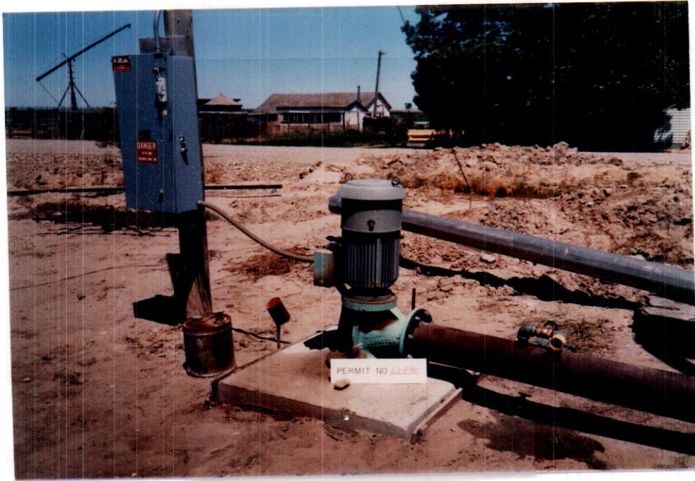
well + 20 HP pump T4N R3W sec 6 NENENE
