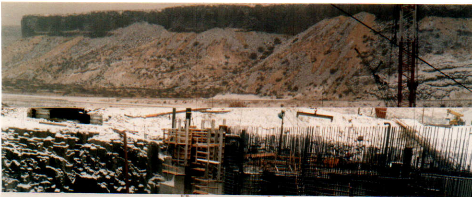
1. Tunnel bifurcation in foreground.
